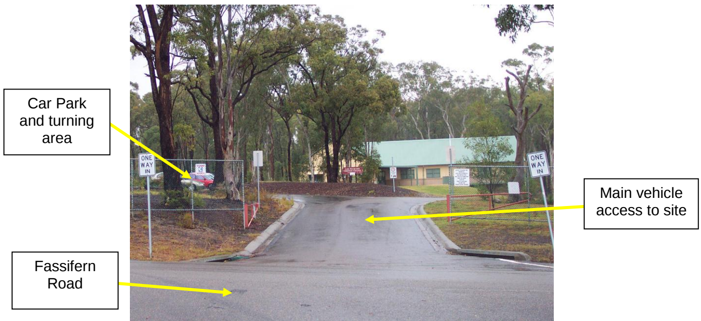
Photograph 01 – View southwest of the subject property from Fassifern Road
